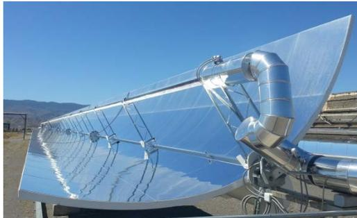
Parabolic trough sandwich mirror
