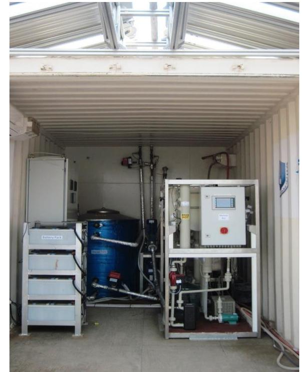
Picture of the portable solar-driven desalination system at KSU
