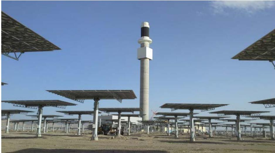
**Figure 10. 110-MW<sub>e</sub> Crescent Dunes Solar Energy Project in Tonopah, Nevada, with ten hours of thermal storage**
