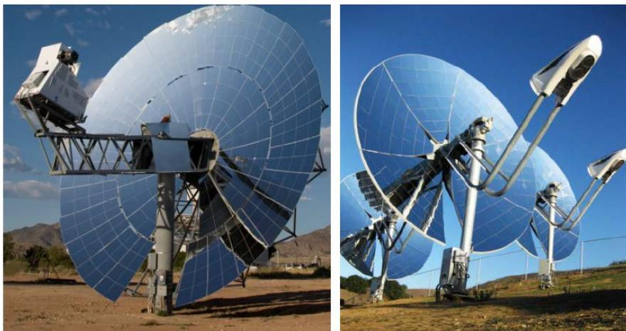
**Figure 12. Two types of dish/engine systems**
