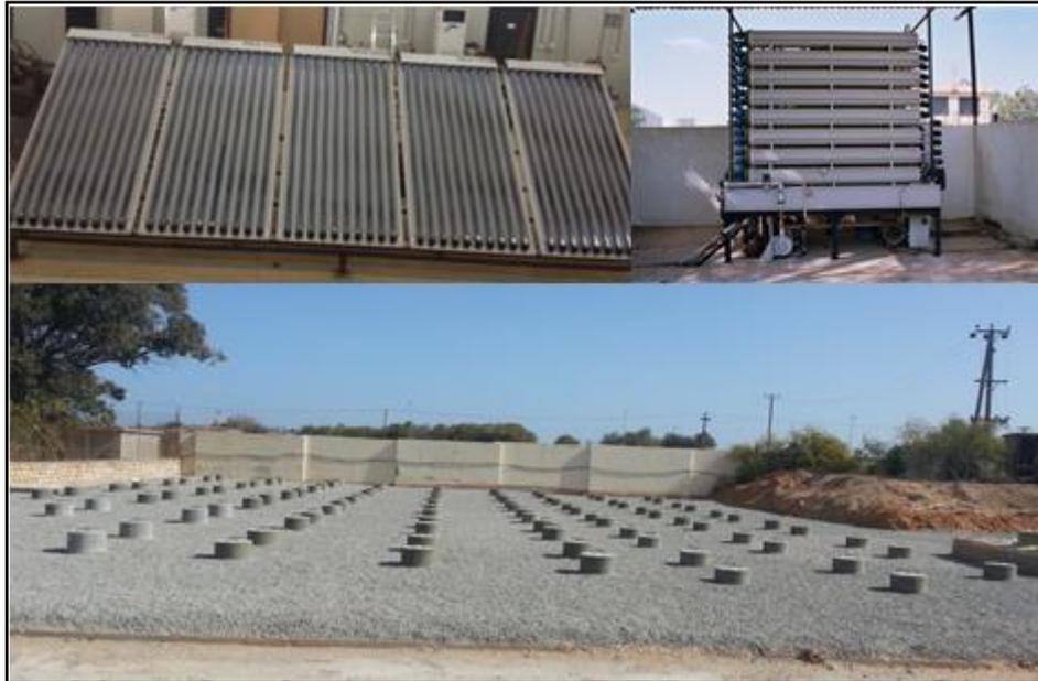
**Figure 17: MSF desalination operated by vacuum tube collector project**
