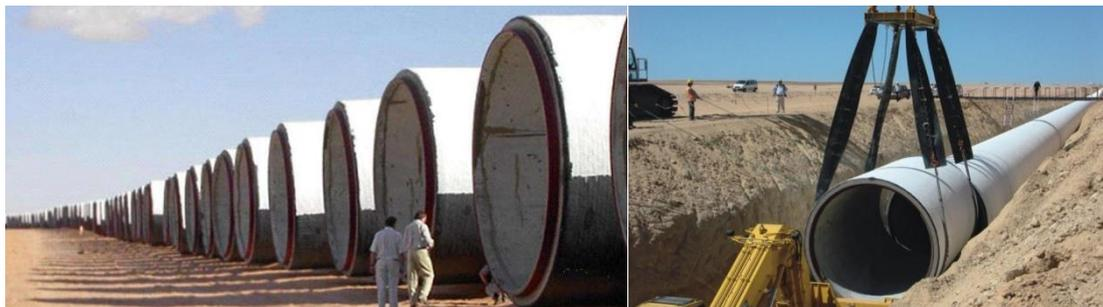
**Figure 8. The Great Man-Made River project – installation of pipelines [18]**
